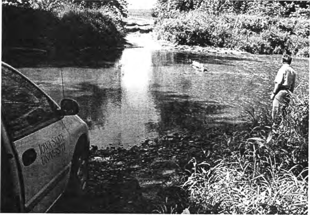
Figure 1. Unvented ford in Iowa constructed with aggregate
