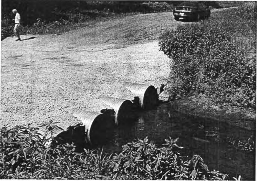
Figure 3. Vented ford with corrugated metal pipes
